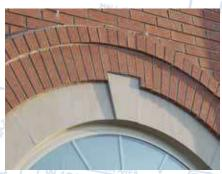
Arches are not easy to construct, especially considering the number of materials which must match and fit together perfectly - structural steel, pre-cast concrete, brick masonry, standing seam metal roof panels, windows and trim/flashings.
