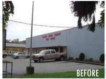
Castles Lumber and Home Center was constructed by us in 1980, with an addition in 1990. The original structure is a pre-engineered building sheeted with metal wall panels and T-III siding.
