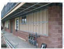
Special attention needed to be given while covering the exterior. All doors, windows and masonry pilasters were carefully coordinated from design through construction in order to work with both existing and new wall panel modules.
