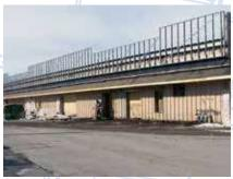
The transformation began by framing custom openings for new doors and windows, constructing a custom canopy out of light gauge metal framing, and wrapping the existing building with stepped parapet walls.
