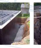
A sloping site required the use of 12 in thick reinforced concrete foundation walls. Integrated piers allowed a pre-engineered building structure to sit atop of the conventionally constructed first floor.
