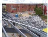
The second floor and exposed portion of building is a preengineered metal building system. Light gauge metal trusses were for dormer and canopy used framing. The roof is standing seam metal, and walls are split-face block masonry and strukturoc metal wall panels.
