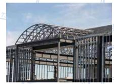
Both barrel roofs are framed with a radius hot-rolled curved truss system. A continuous curved valley was framed and flashed where the barrel roof meets the main roof.
