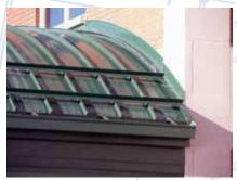
Special conditions, such as flashing the curved canopy roof to the brick and pre-cast concrete veneer, required special attention from the design phase through completion.
