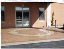
Attention to detail can also be seen in the stamped concrete at the main entrance below the drive-through canopy. A stamped brick herringbone pattern is used in conjunction with a circular keystone design.
