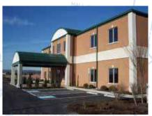
Both barreled roofs are identical with their matching standing seam metal roofs and dryvit covered curved gables. Pre-cast concrete is used extensively throughout the exterior.
