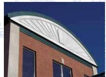
Special attention is given to the smallest details. Both curved gables are covered with dryvit in a butter-knifed fan pattern emanating from a raised keystone.
