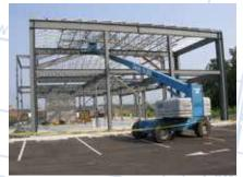
The hybrid structural system combines the advantages of a preengineered system and conventional steel framing. Second floor structure is conventional bar joist/metal deck; while the roof framing is a combination of pre-engineered frames and purlins with light-gauge metal trusses to form the hip roof.
