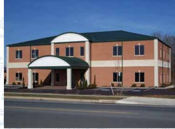
This 13,235 sq.ft., two story medical facility was a challenging design/build project. The hybrid structural system and foundations are designed to accommodate sensitive medical equipment, and the materials used were chosen in order to satisfy a perfection-oriented owner.
